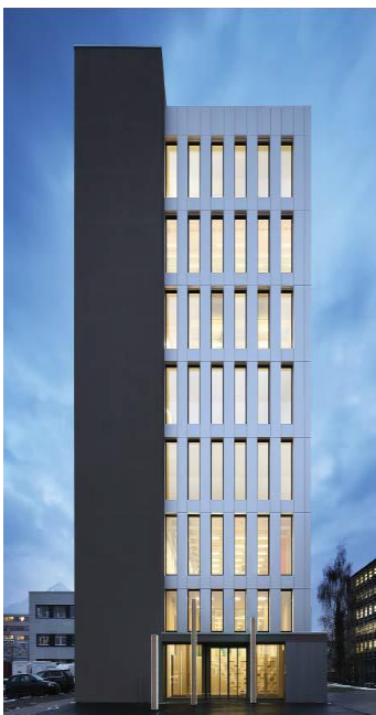
Life Cycle Tower, Dornbirn, Autriche Bureaux, R+7 Structures mixtes Bois/Béton
