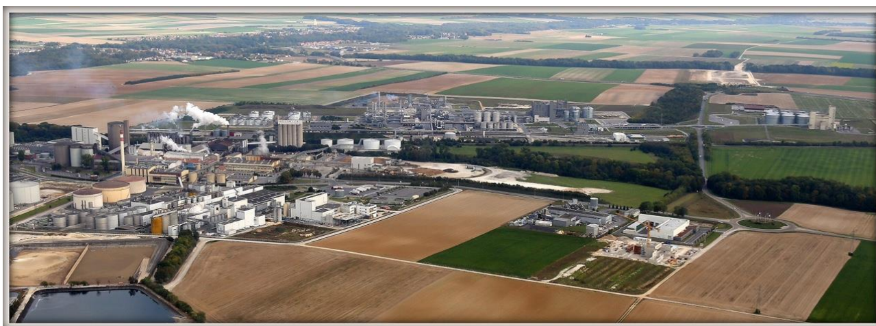
Bioraffinerie de Bazancourt Pomacle - (credit photo D.DUTARTRE)
